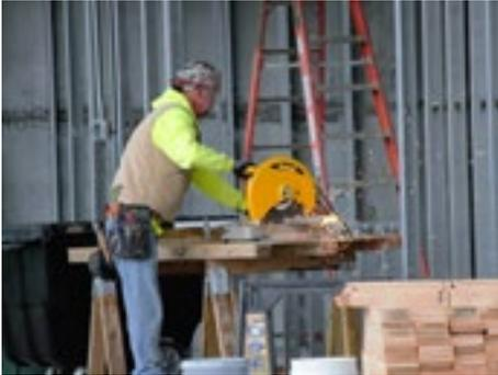
**Cover Photo:** A member of the Indiana/Kentucky/Ohio Regional Council of Carpenters cutting down steel studs for the the new Carpenter's Training Center in Hobart, IN. Hasse Construction is the General Contractor on the project and Ron Holsclaw is the General Superintendent.
